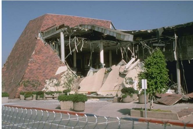
**Figure 7.12:** Partial building collapse due to failure slab-column connections after the 1994 Northridge Earthquake (photo by NOAA/NGDC, J. Dewey, U.S. Geological Survey).
