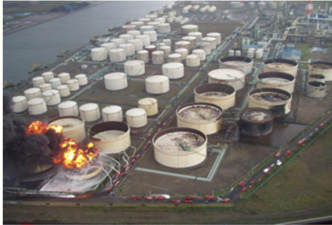
**Figure 2.8:** Oil storage tank damage due to long-period shaking after 2003 Tokachi-Oki (Photo Credit: <http://mycommittees.api.org/standards/cre/scast/>)
