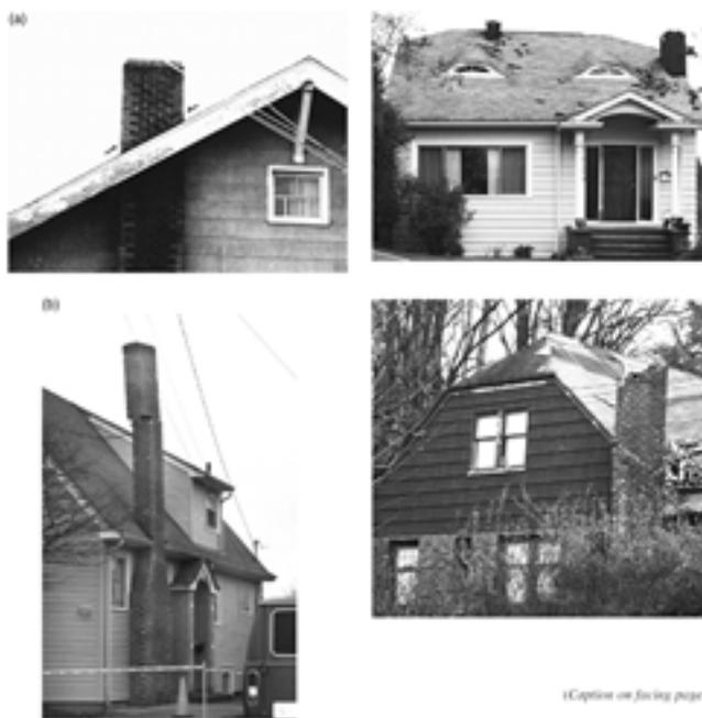
**Figure 2.7:** Localized chimney damage (in West Seattle) after 2001 Nisqually (Photo Credit: Booth (2004))
