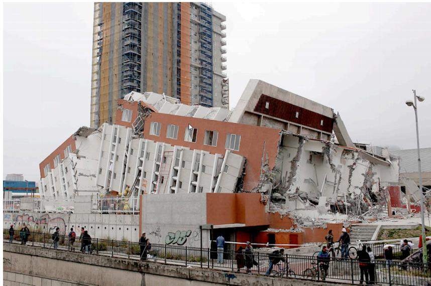
**Figure 2.3:** Collapse of the Alto Rio building after the 2010 Maule Earthquake (Photo Credit: USGS Open-File Report 2011-1053 v1.1) (2011).
